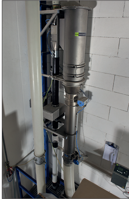
Installation example: GF 4000 metal separation systems installed in vertical pressure pipes. (old version)
